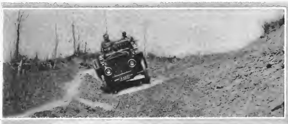
Typical Road Almost Anywhere Between Washington and Richmond.
